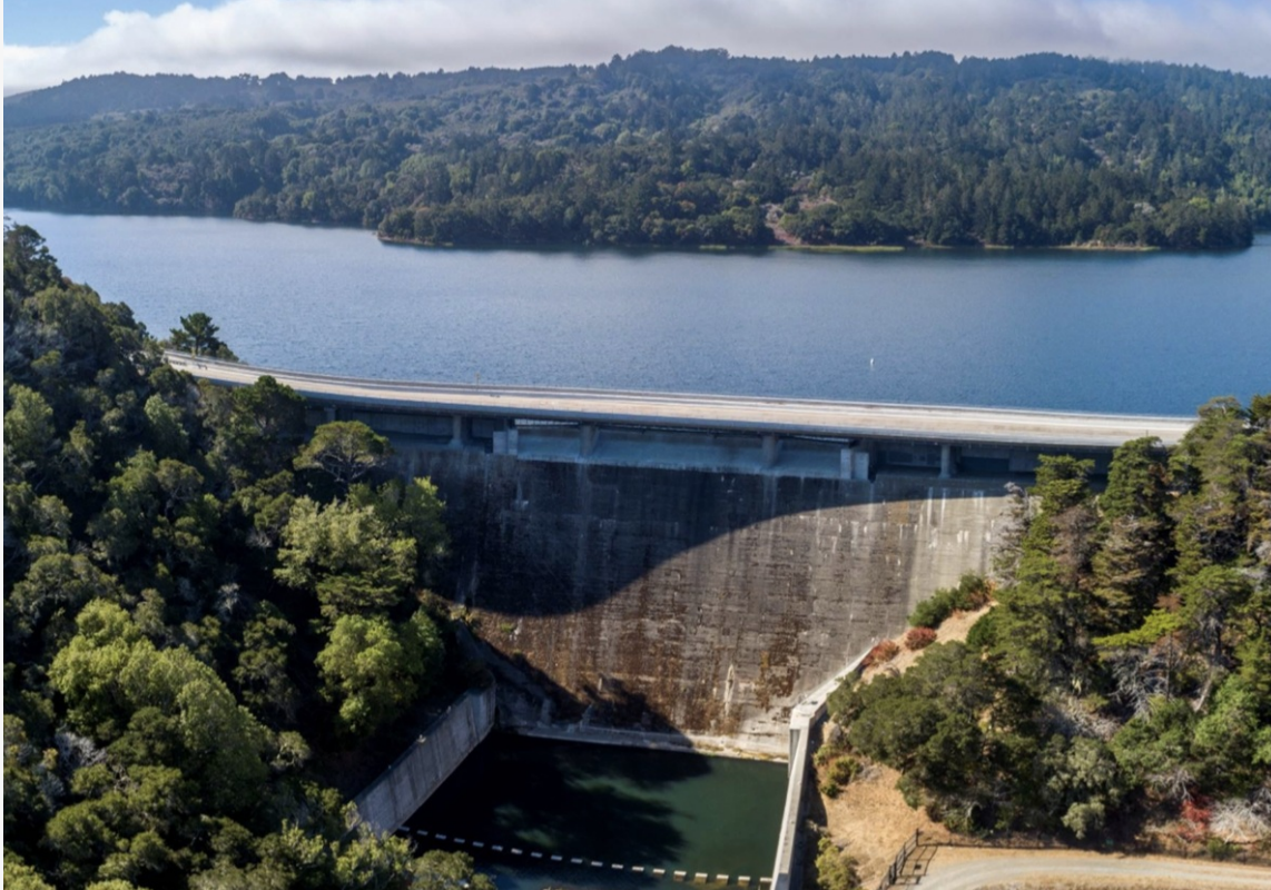
Built in 1886-89, Lower Crystal Springs Dam is still in use today (Photo credit: SFPUC)
