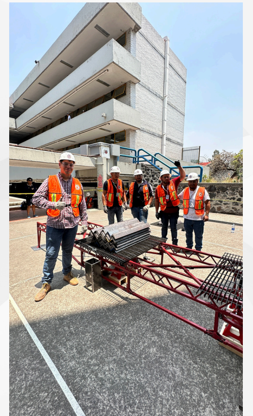
Completing vertical load test at the Michoacana University of San Nicolás de Hidalgo
