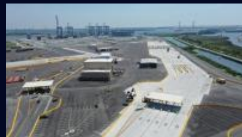
Hugh K. Leatherman Terminal Phase 1 Construction Project
