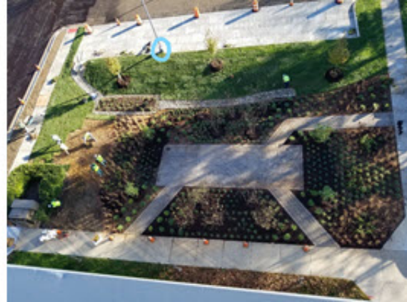
The east parking lot, before and after. It now features a bioretention zone for water drainage, as well as permeable pavers and precast porous concrete slabs.
