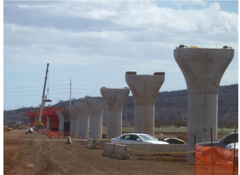
Possible Site Visit: Rail Project in Kapolei
